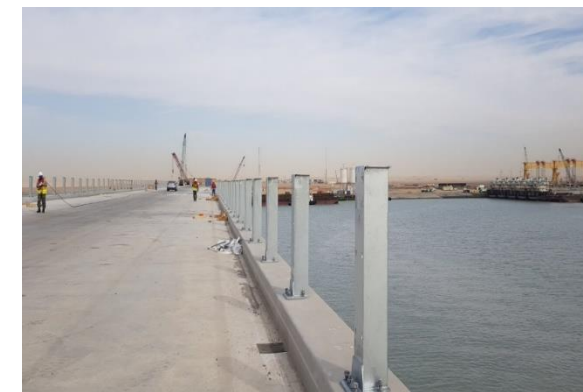
6. Rail installation completed
