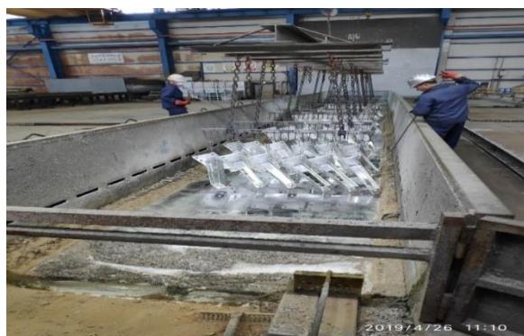
3. Zinc Hot Dip Galvanizing
